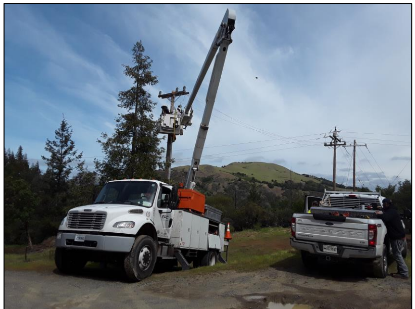
Photo 4: PG&E Coordination under line on Eldridge Grade.
