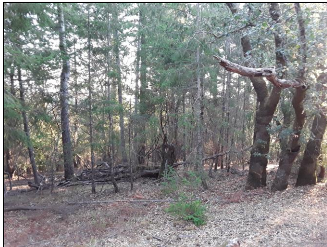
Photo 25: Fuelbreak Construction at Taylor Trail Before
