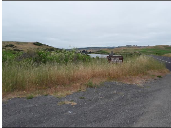
Photo 17: Nicasio Reservoir Before
