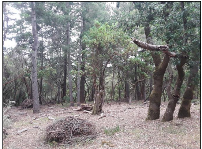
Photo 26: Fuelbreak Construction at Taylor Trial After
