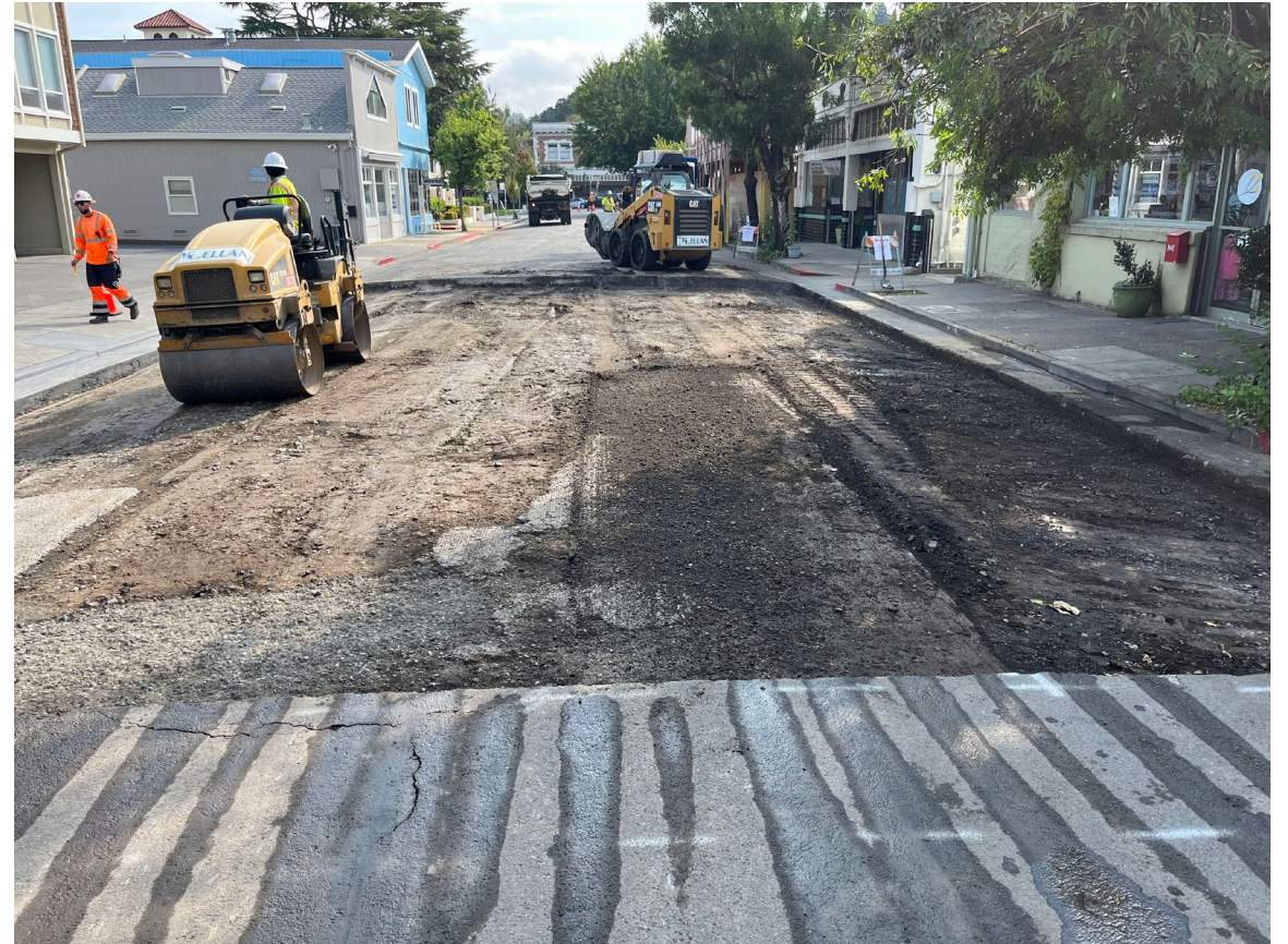
138 Tunstead Avenue – 2,400 square feet of 2"-8" thick asphalt paving
