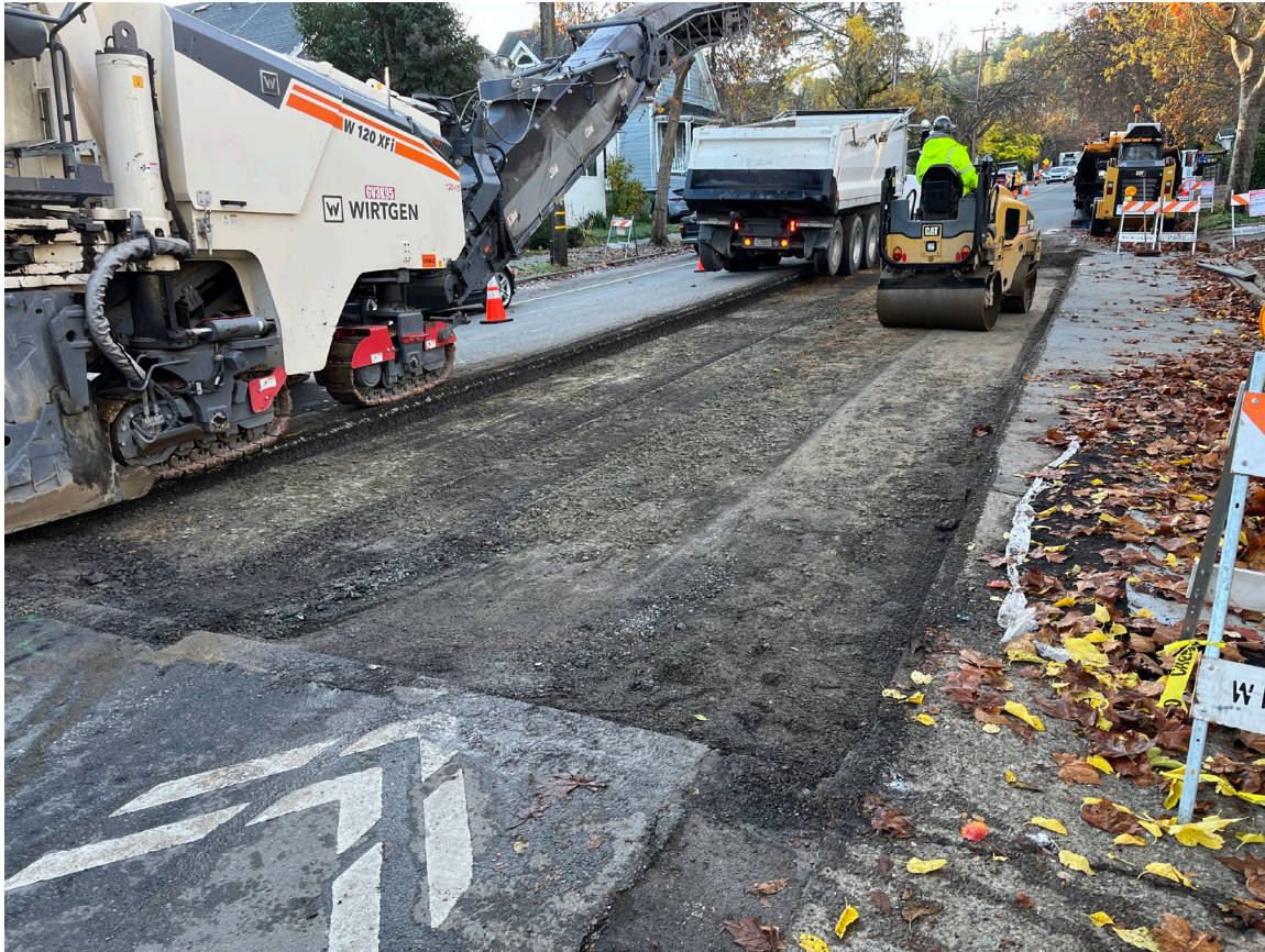
343 D Street – 2,412 square feet of 2"-10" thick asphalt and concrete paving
