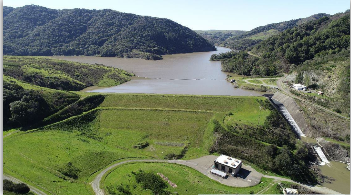
Soulajule Dam & Pump Station
