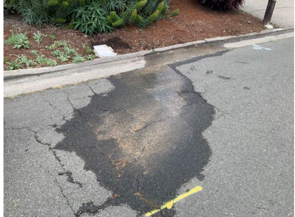
District Service Leak
