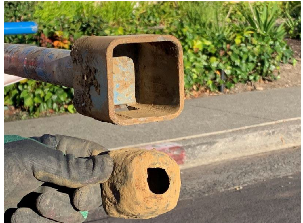
With Corroded Operating Nut
