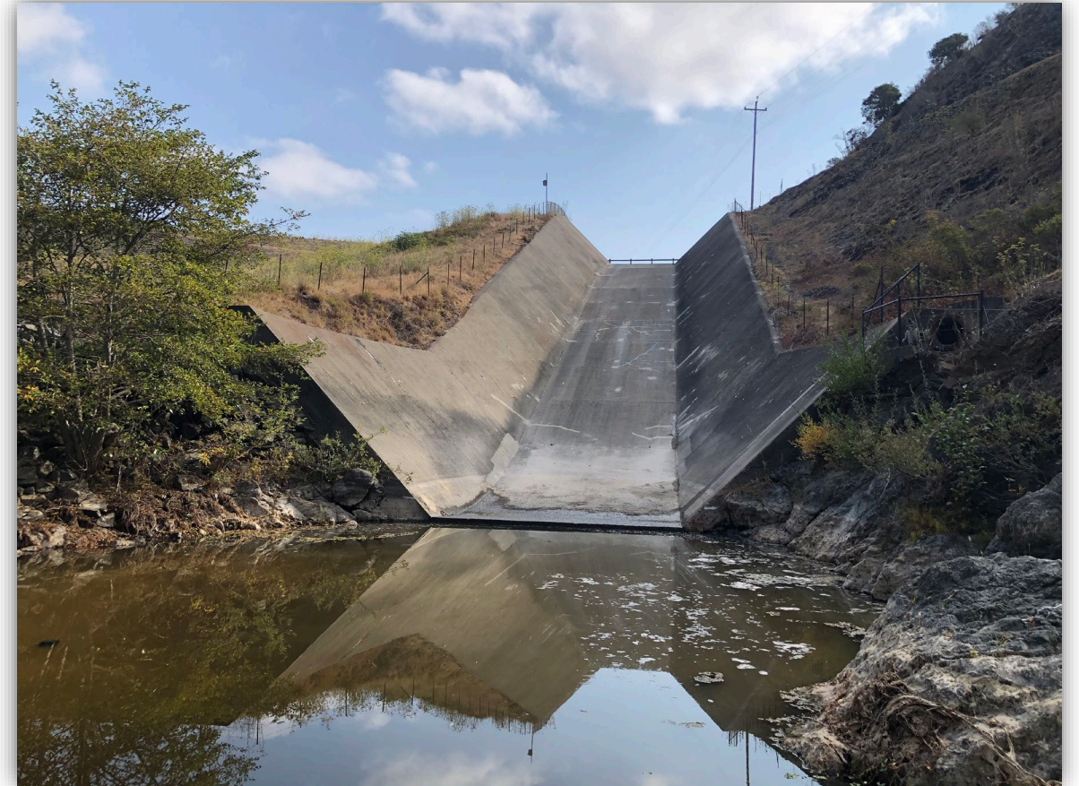
Spillway of Seeger Dam, Nicasio Reservoir
