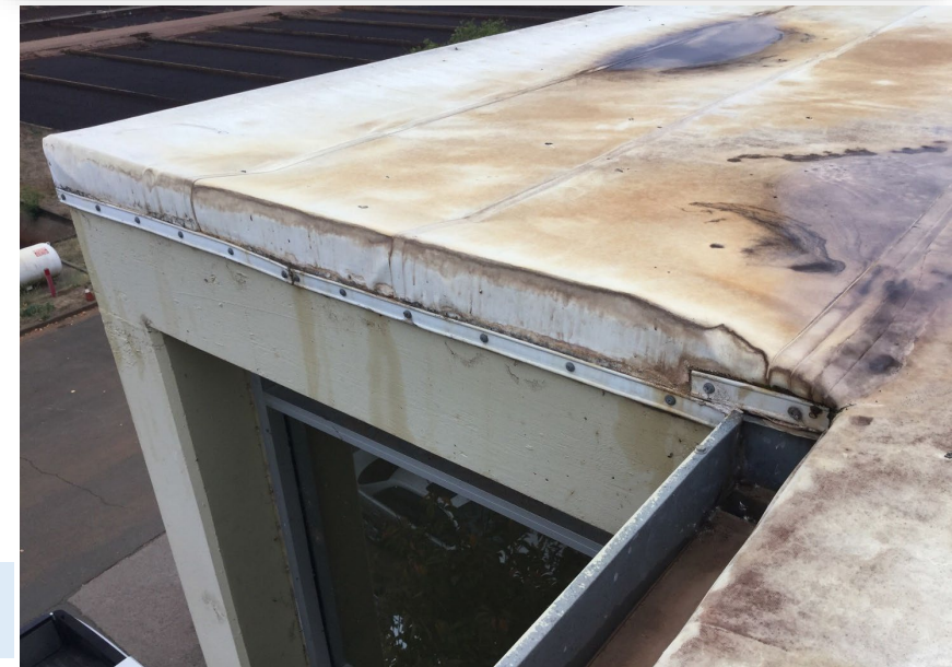
San Geronimo Treatment Plant Roof
