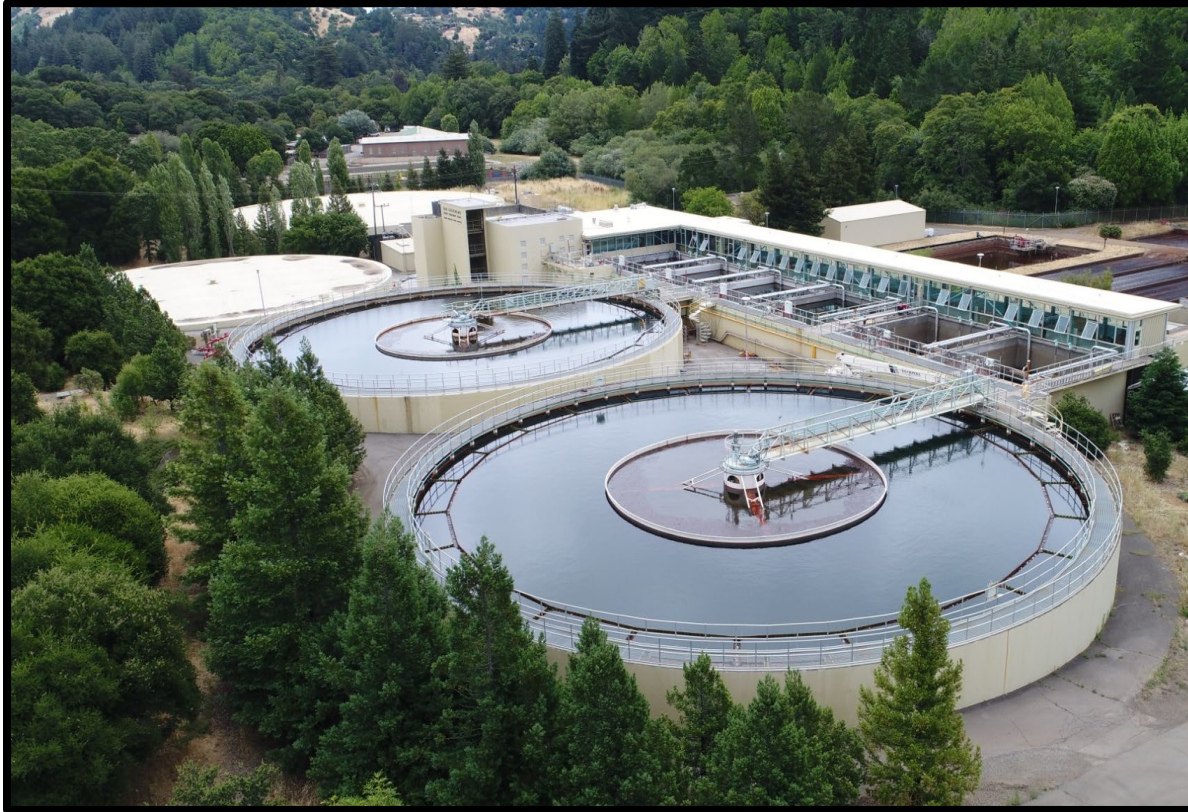
Existing Clarifiers lack lateral resistance, SGTP Clarifiers
