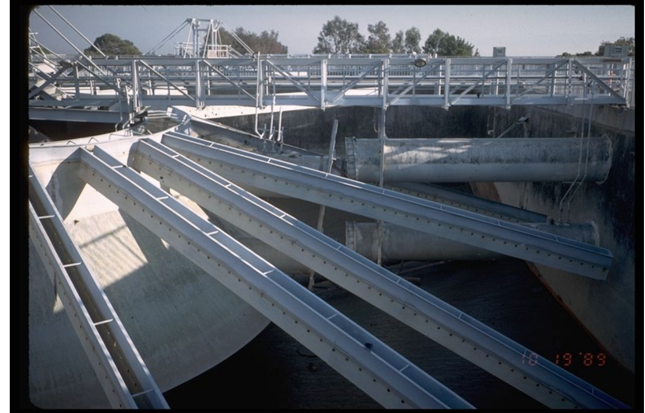
Rinconada WTP Clarifier After Loma Prieta EQ,
