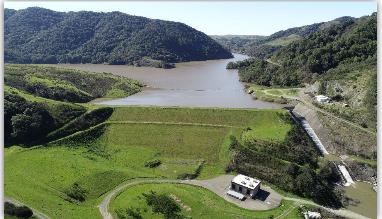
Soulajule Dam & Pump Station
