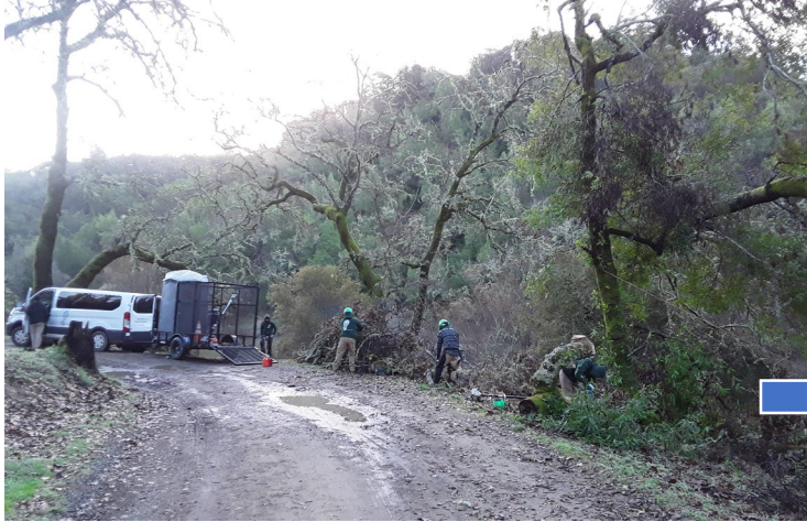
Fire road brushing and fuelbreak maintenance
