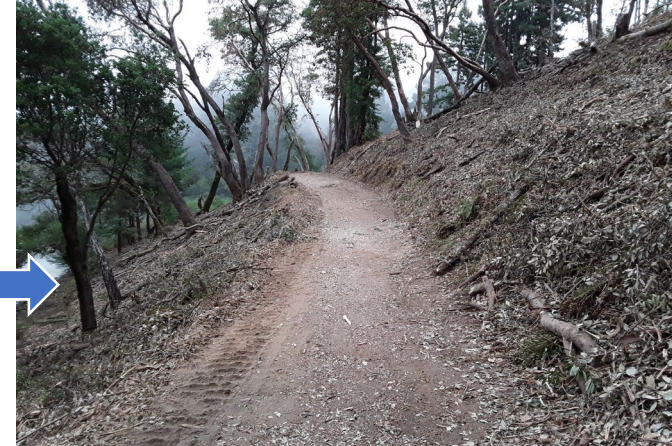
Lake Lagunitas Forest Restoration
