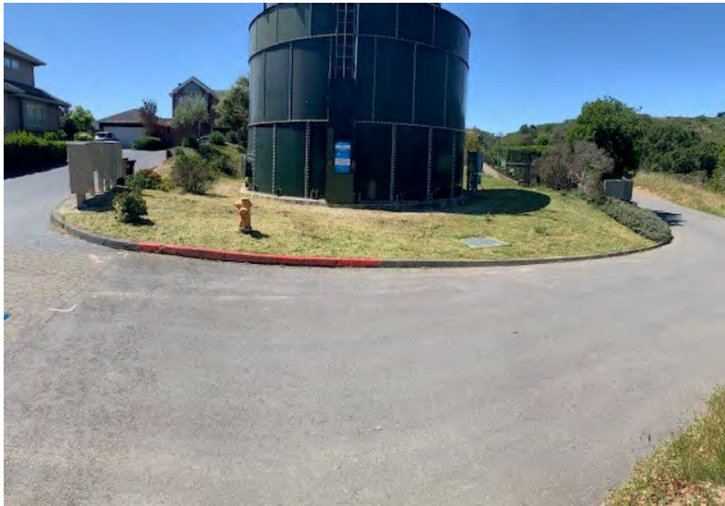
Fairview Park Tank Before and After
