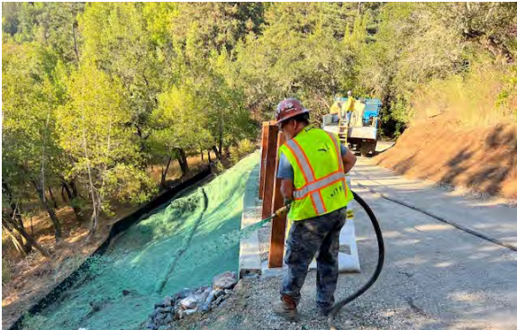
Worn Springs Rd retaining wall
