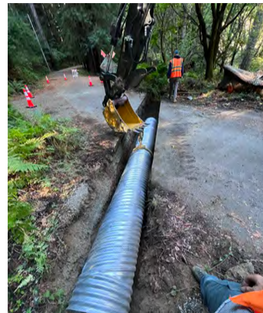
Culvert replacement
