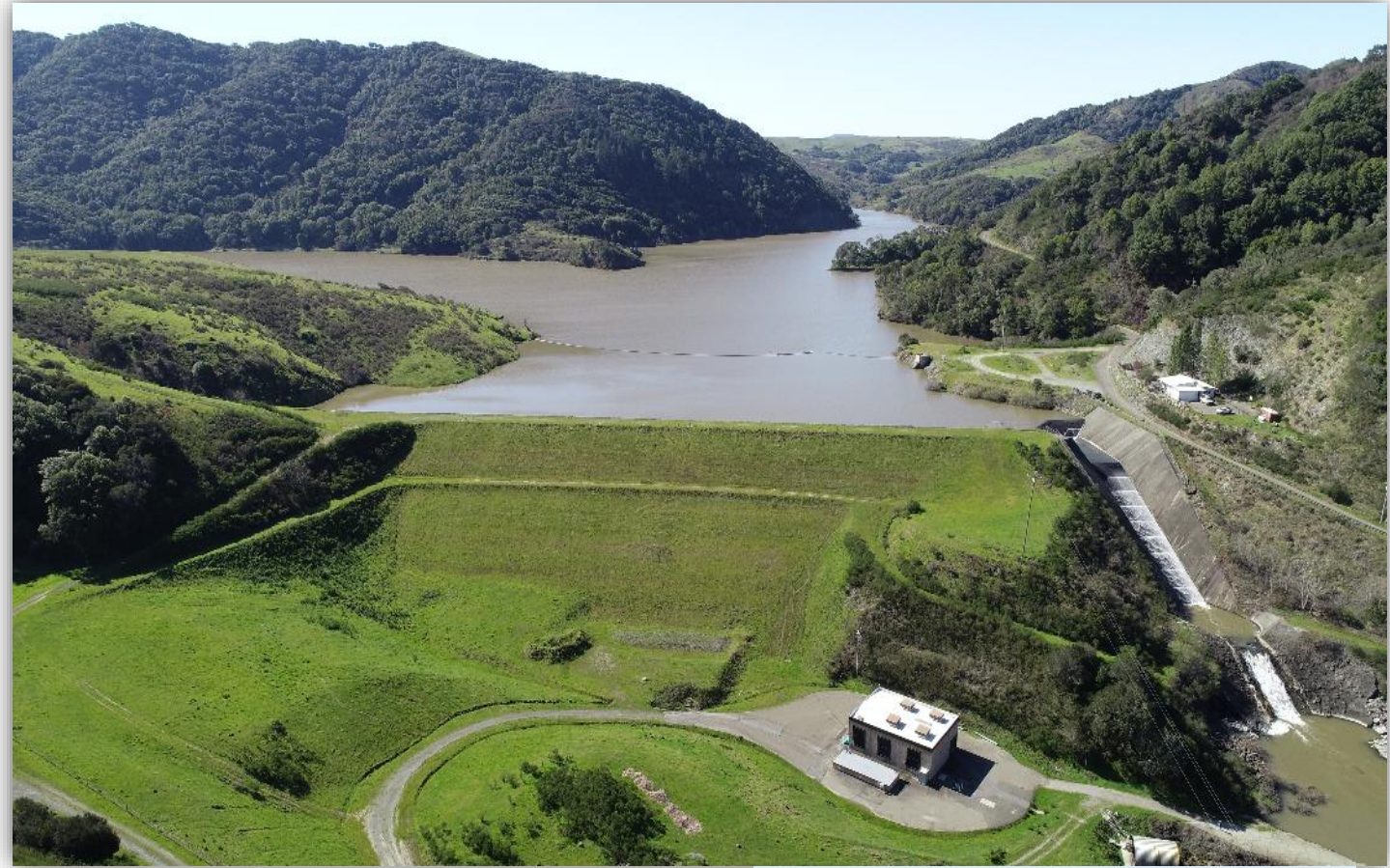
Soulajule Dam & Pump Station
